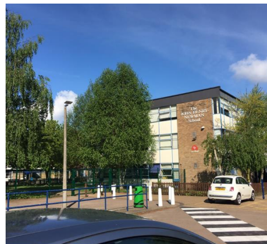
The current Main Block which will be demolished in 2024
